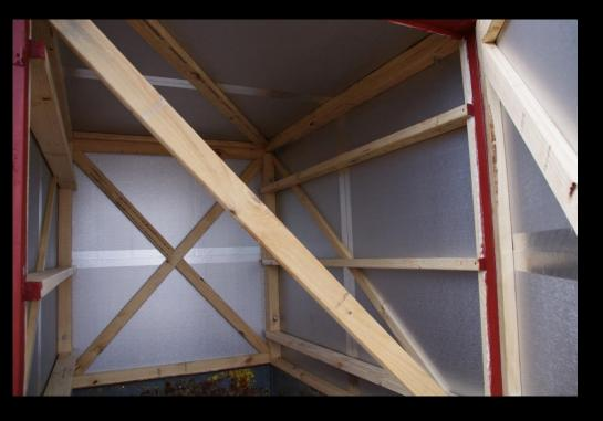
I worked out a framework to build the box so it was sturdy and could be assembled and pulled down on my own.
